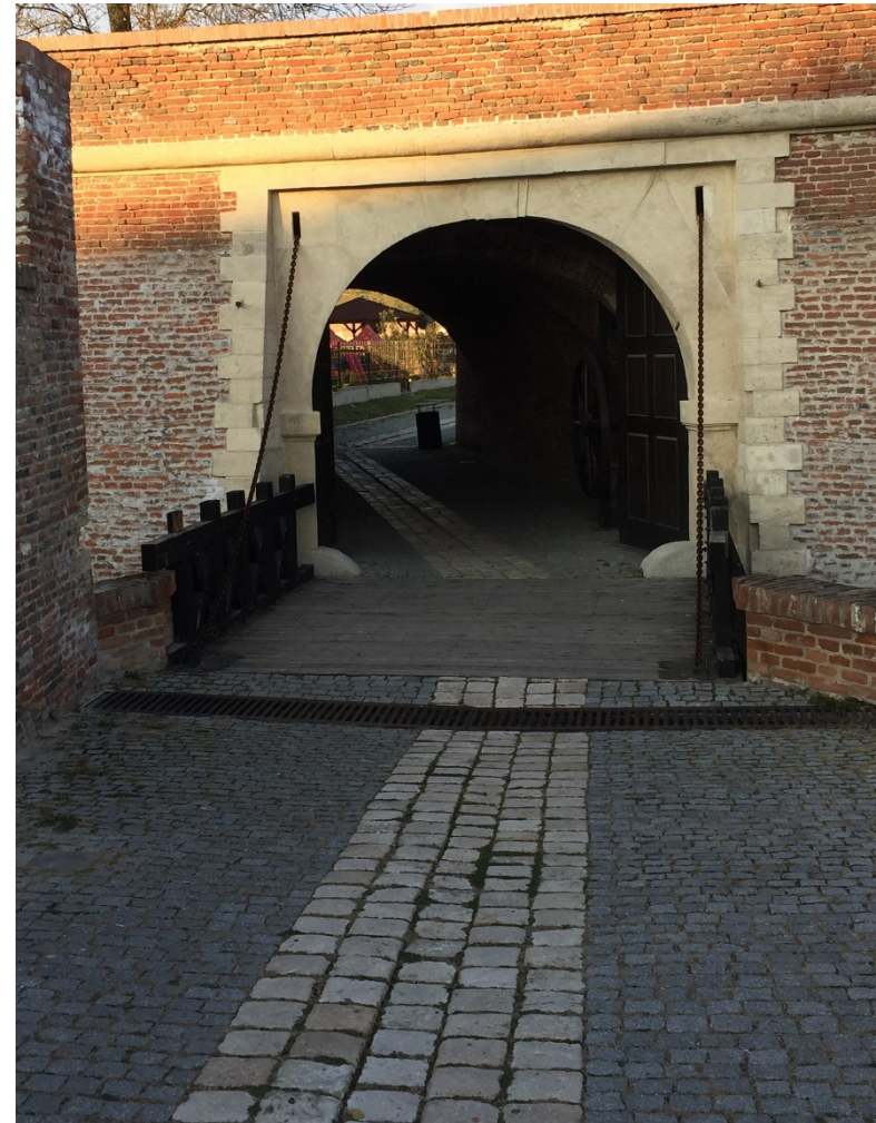
Restored Roman Roadway, Alba Iulia, Romania
